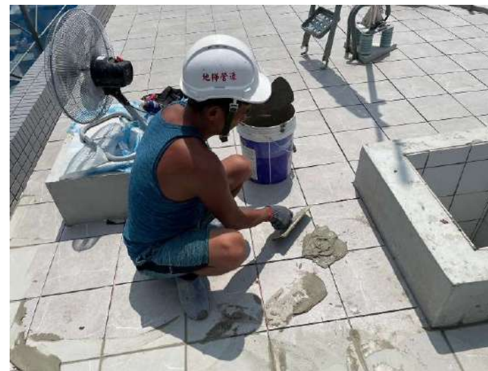
RF水箱及屋頂版磁磚填縫
