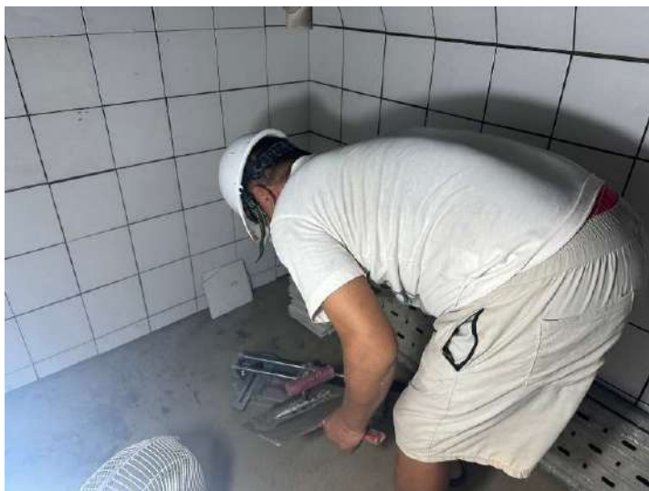
R3F水箱磁磚鋪貼
