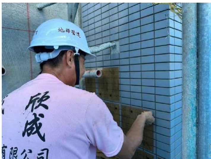
5F南側外牆磁磚施作
