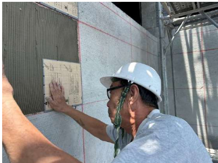
11F北向外牆磁磚施作
