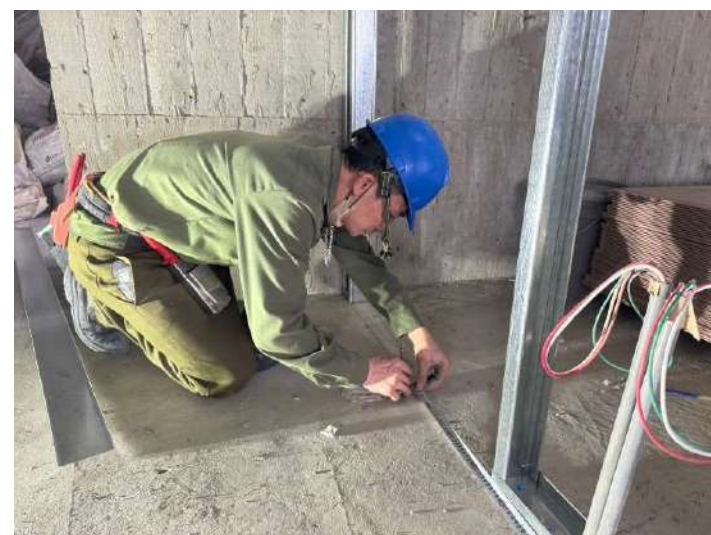
9F輕隔間骨架施作
