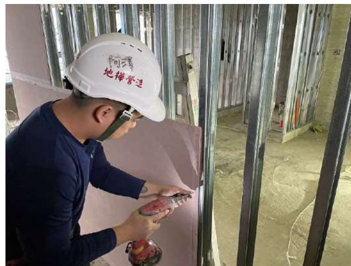
9F輕隔間單板施作
