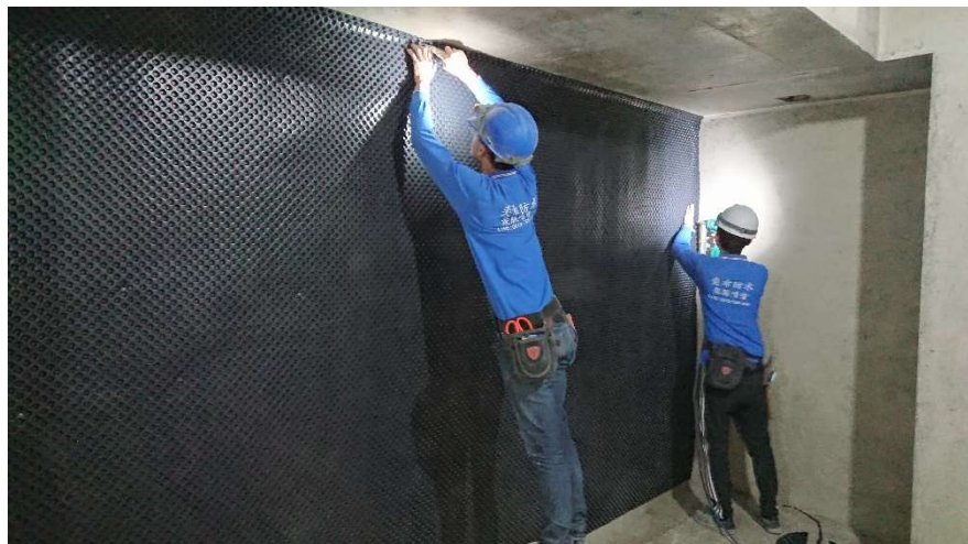
B1F 導水版施作
