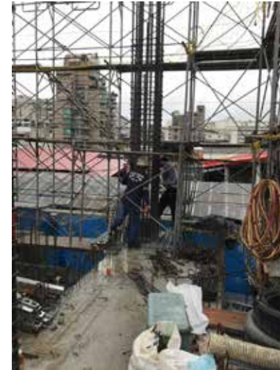
5F柱筋綁紮
