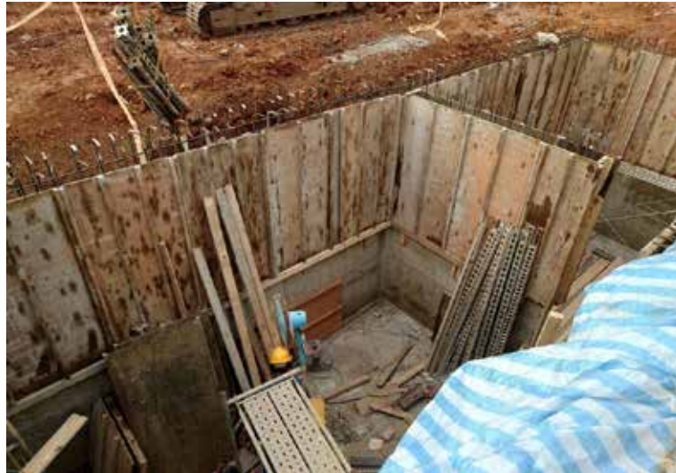
滯洪池拆模及上部立牆模
