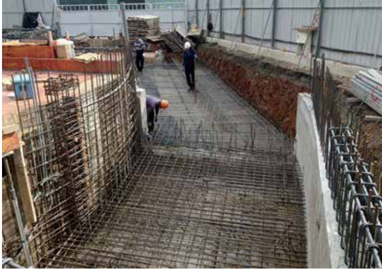
車道版筋綁紮
